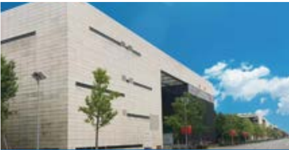
Shanghai Telecom Data Center
