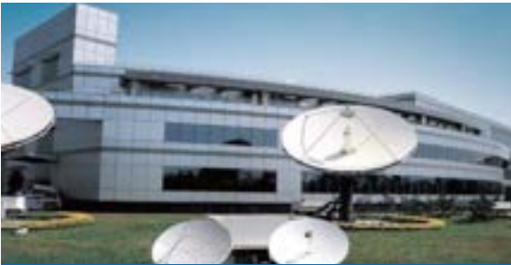
Shanghai Securities Waigaoqiao Earth Station
