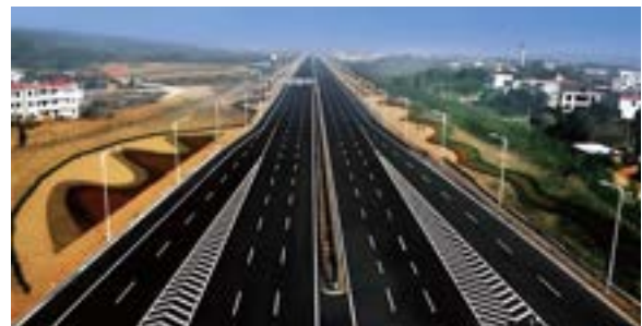
Ruili to Menglian Expressway Electromechanical Project
