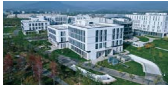
Peking University Biomedical Imaging Technology Cluster Large Facility
