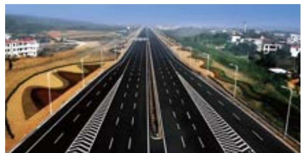
Ruili to Menglian Expressway Electromechanical Project
