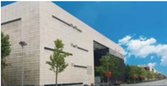
Shanghai Telecom Data Center
