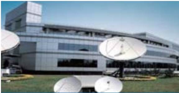
Shanghai Securities Waigaoqiao Earth Station
